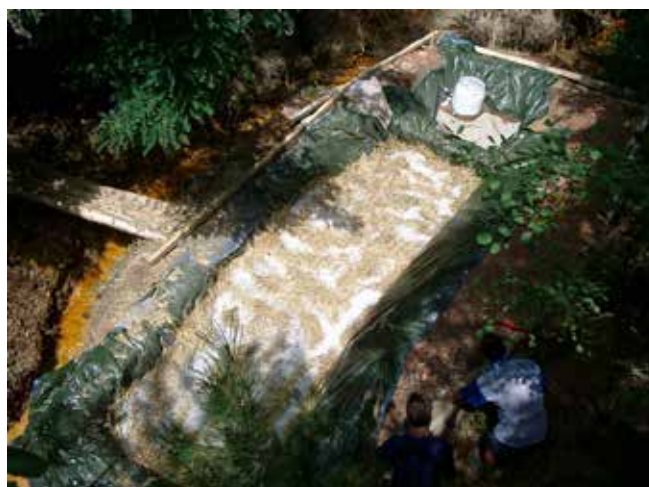
Fig. 10. Treatment of acid mine drainage by means of permeable reactive multibarrier in the Kurilo deposit
